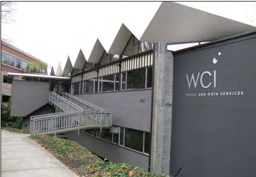
Figure 42. Below, 1945 Yale Place North (1960), Seattle. Designed by A.O. Bumgardner, Modern-style example.
