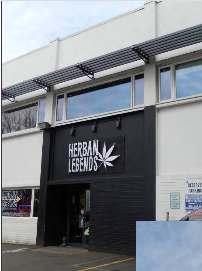
Figure 29. Left, detail of secondary building entrance, with steel brise soleil across the top of the second floor window heads. Steel sash windows have been replaced with vinyl. Norman brick infill panels have been painted black and white, and the steel brise soleil has been painted black.
