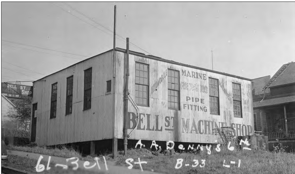
Figure 8. Below, King Co. Tax Assessor's photograph, 1937 of the previous (ca. 1914) machine shop building on the site of the subject building. (Puget Sound Regional Archives).
