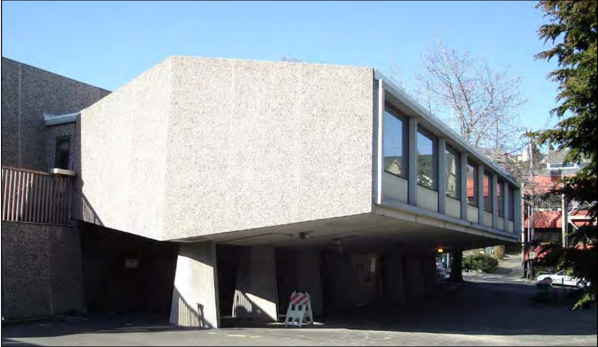
Figure 41. Above, 157 Roy Street, (1963), Seattle. Designed by Harmon, Pray & Detrich, Modern-style example.
