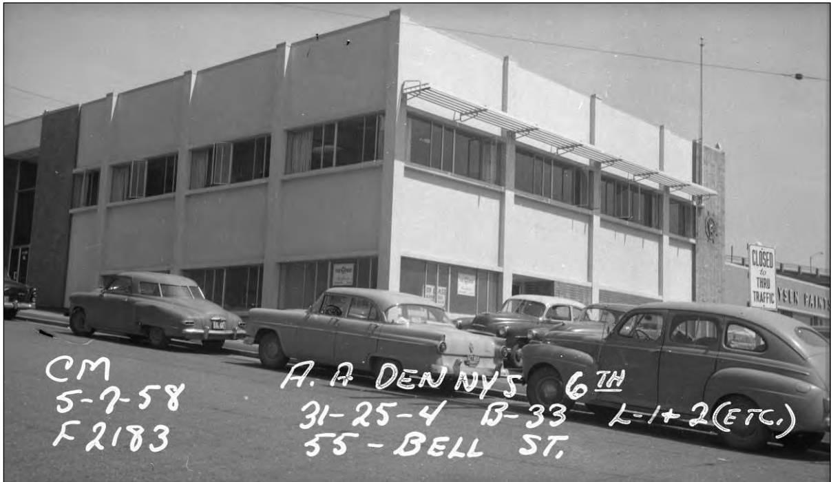
Figure 15. Above, King Co. Tax Assessor's photograph of the subject building, 1958 (Puget Sound Regional Archives).
