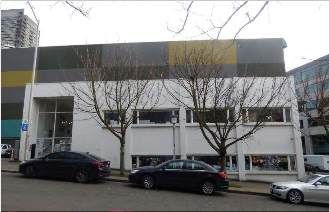
Figure 25. Above, looking south at the primary north façade, which faces Bell Street. Original steel sliding windows have been replaced with vinyl in a different configuration and the contrasting Norman brick entry pilasters have been painted to match the remainder of the concrete building. The multi-colored six story building rises behind.
