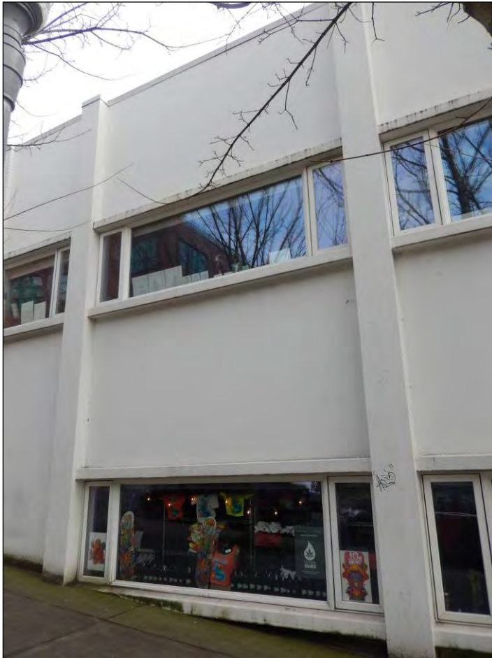
Figure 27. Left, detail of painted concrete pilasters and spandrels, and ribbon windows on primary north façade. Note cast window heads and sills.
