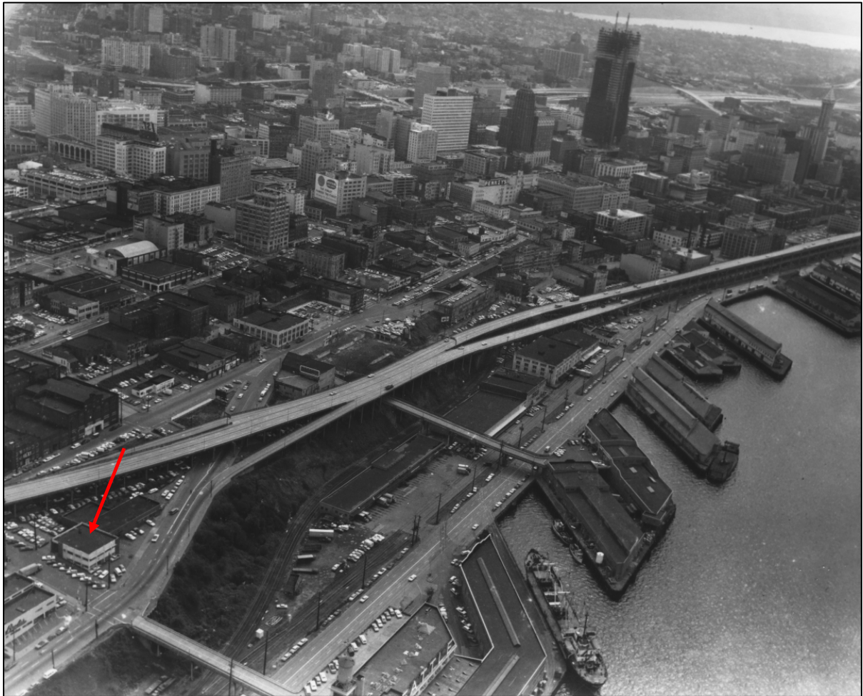
Figure 11. Above, an aerial view of the area, looking southeast, 1968. The subject building is noted with a red arrow. (Seattle Municipal Archives Image #33047)
