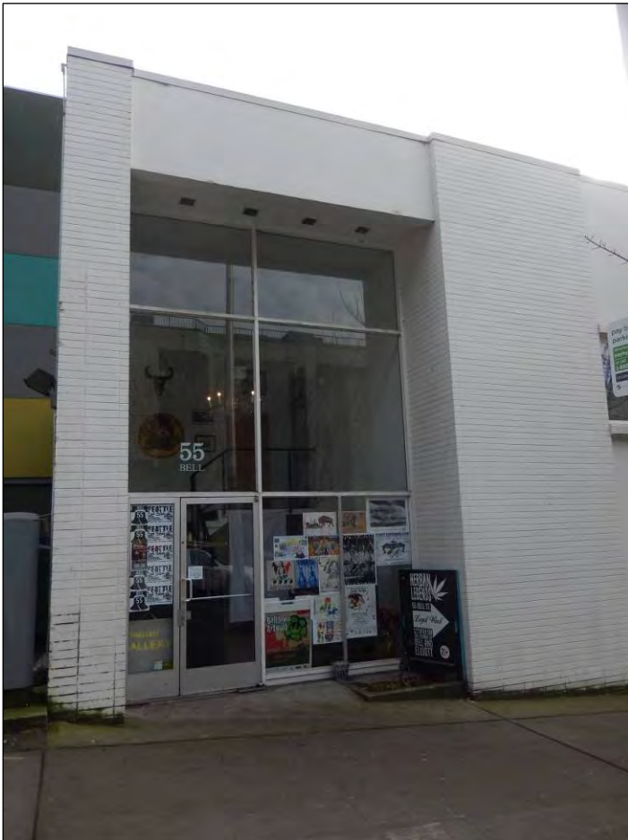
Figure 25. Above, looking south at the primary north façade, which faces Bell Street. Original steel sliding windows have been replaced with vinyl in a different configuration and the contrasting Norman brick entry pilasters have been painted to match the remainder of the concrete building. The multi-colored six story building rises behind.
