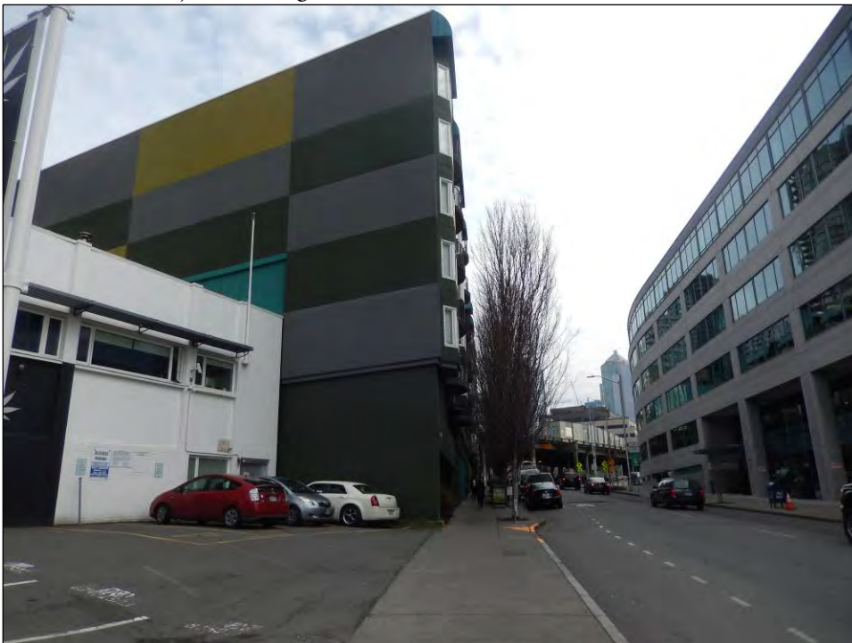
Figure 20. Below, looking south toward the Alaskan Way Viaduct along Elliott Avenue. The subject building is on the left.
