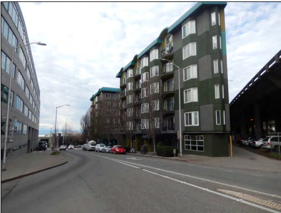
Figure 22. Below, looking north from the intersection of Elliott Avenue, Western Avenue and the ramp to Route 99 southbound, toward the subject building which is hidden behind the six story building to the right.
