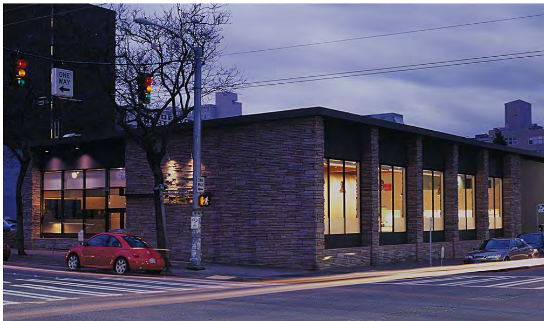
Figure 46. Below, 2333 3 rd Avenue, (1951), Seattle, demolished.
