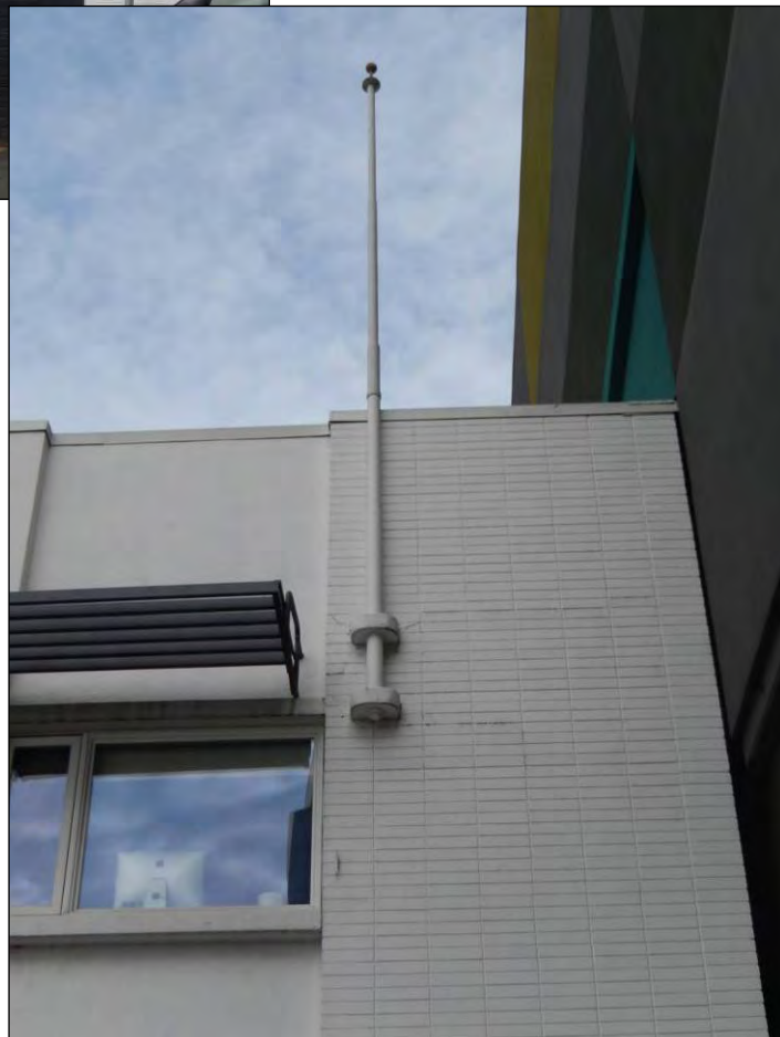
Figure 30. Below, flag pole mounted on the painted Norman brick veneer, ribbon window, and brise soleil detail on the left.
