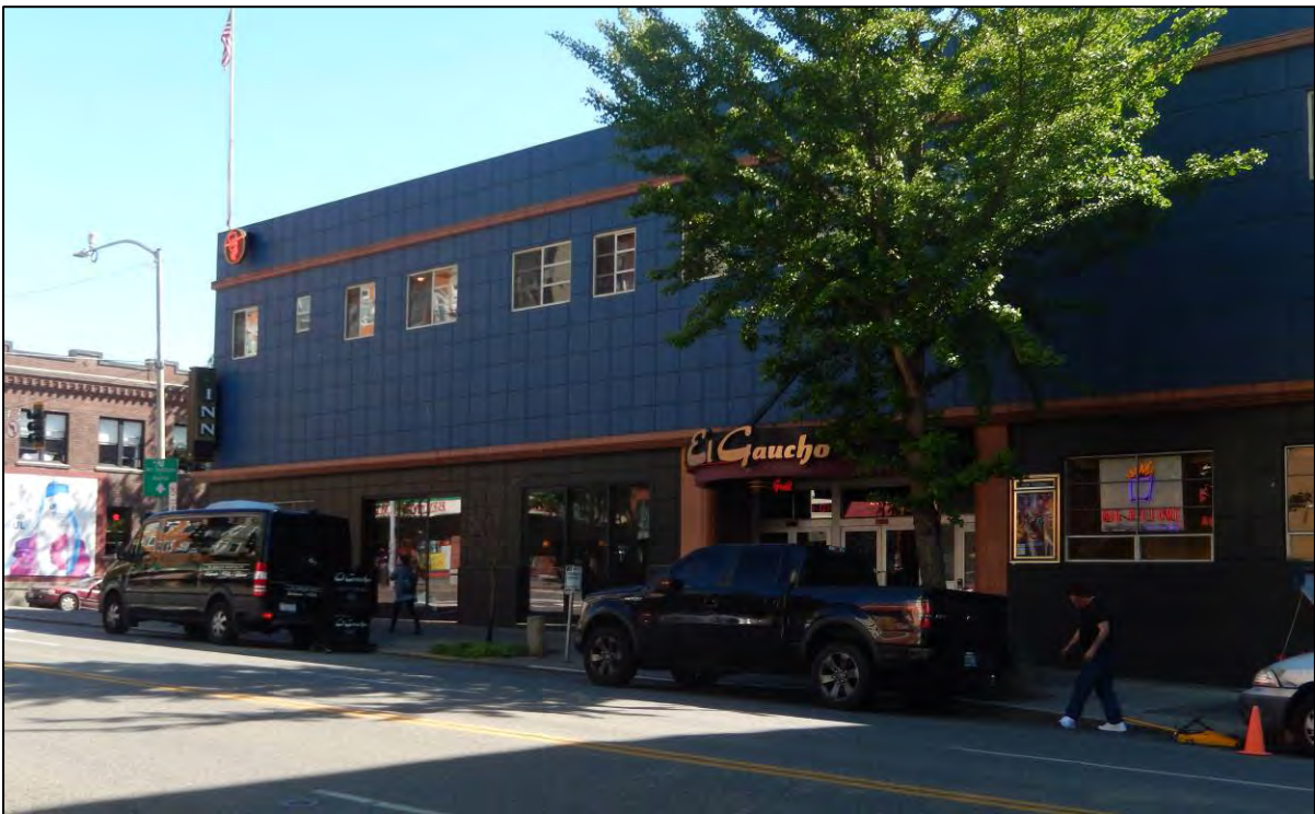
Figure 36. Below, Sailor's Union of the Pacific (1954), 2502 1 st Avenue, City Survey Category 1.
