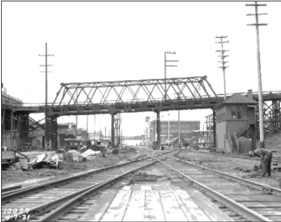
Figure 7. Above, view looking north along Railroad Avenue at the Bell Street Railroad Trestle, 1931. (Seattle Municipal Archives, Image # 4870)
